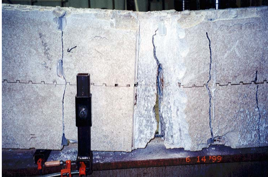
Figure 5c Typical Failure Mode for the Long-Span ICF Flat Lintel (4x24 specimen with foam removed at primary failure location)
